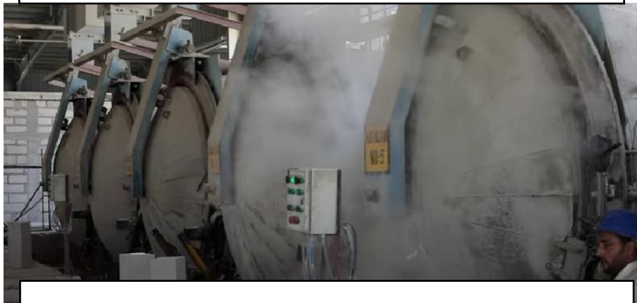
Steam Curing Process (Autoclave Reactor)
